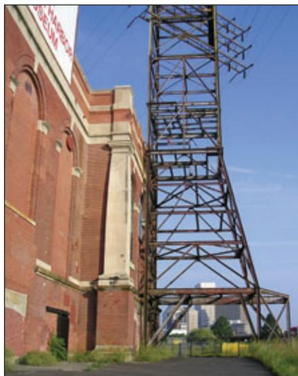
Fig. 4: Steel latticework can trap moisture, causing accelerated corrosion.
